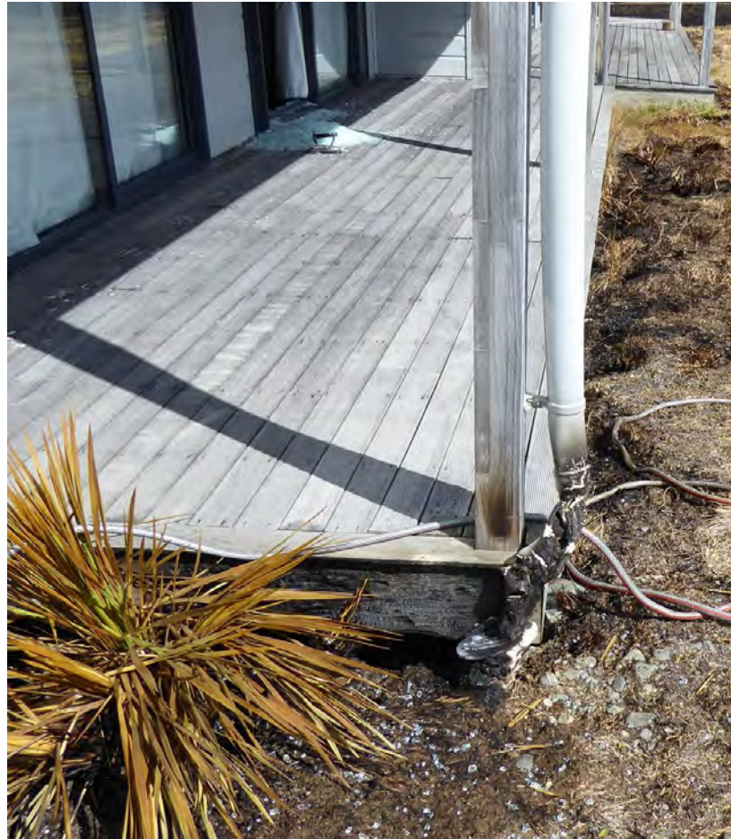
Figure 17: Example of how vulnerable wooden decks are to being ignited via direct flame, ember attack or radiant heat exposure
